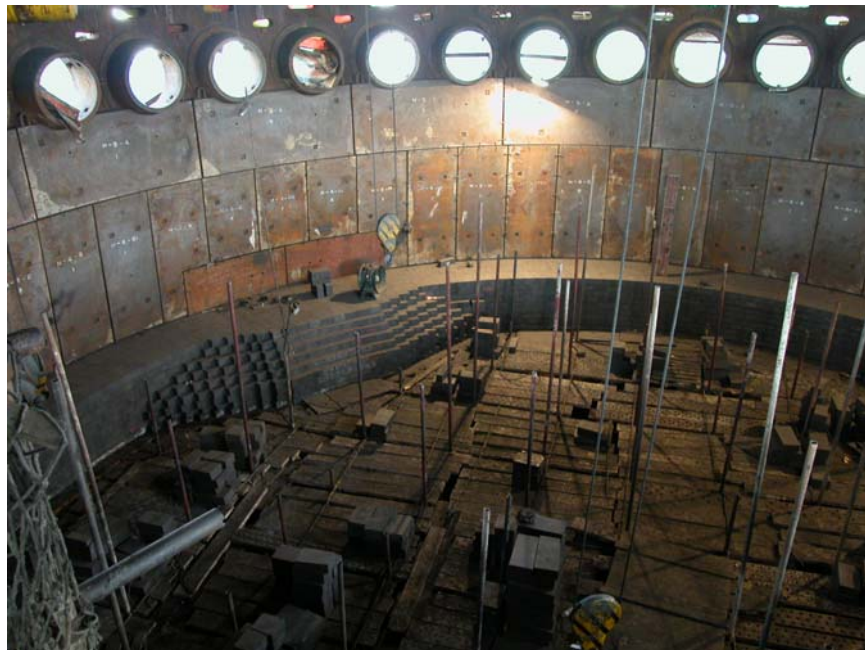
Figure 10 - Installation of the GrafTech International lining in Baosteel's No. 4 Blast Furnace
