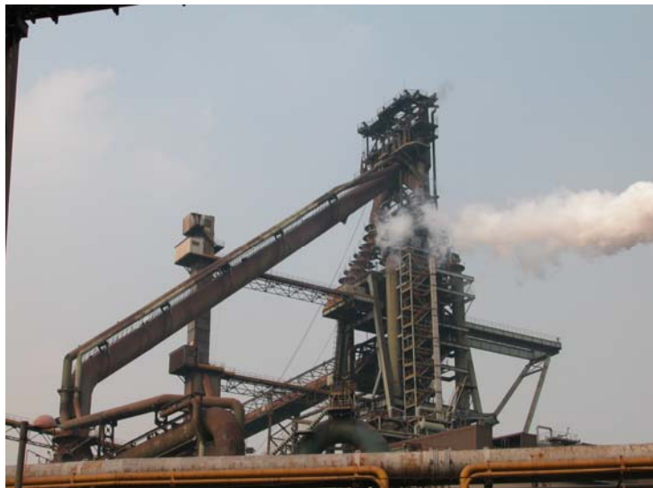
Figure 9 - Baosteel No. 3 Blast Furnace
